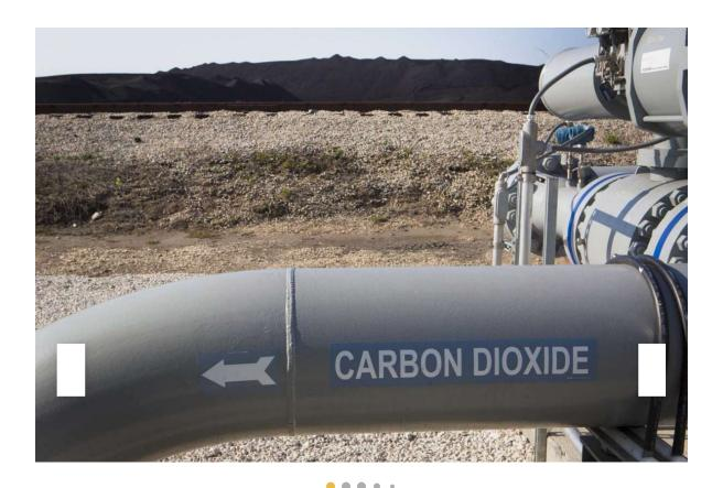
WA Parish plant infrastructure at Fort Bend County. NGR Energy and JX Nippon Oil & Gas Exploration Corporation have built the Petra Nova Carbon Capture Project. The project is a commercial-scale carbon capture system that captures carbon dioxide in the processed flue gas from an existing unit at the WA Parish power plant. Tuesday, Dec. 20, ...
